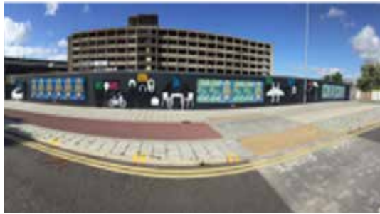
Cattle Market Road Demolition
