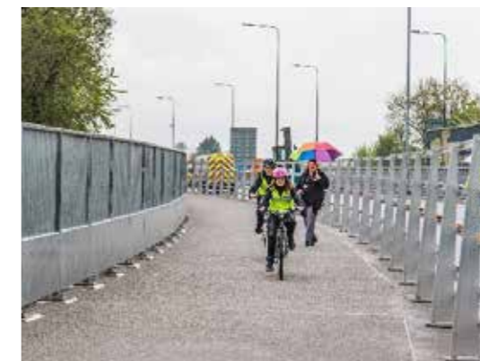
Bromley Heath Viaduct, South Gloucestershire
